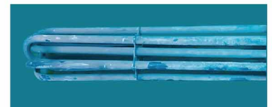
Status before cleaning
