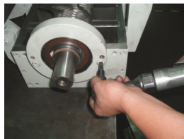
Picture 6-13: Installation of Fixed Blades and Rotating Blades 2
