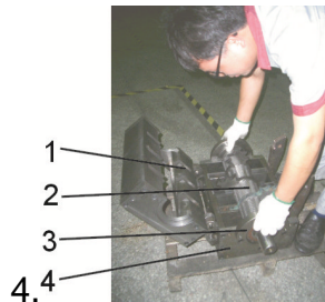
Picture 6-3: Installation of Bearing and Blade Rest 3
